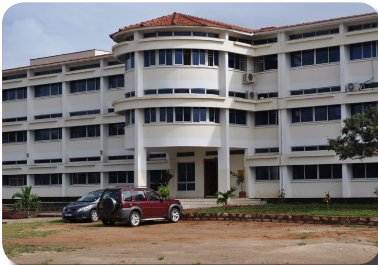
The New Administration Block
