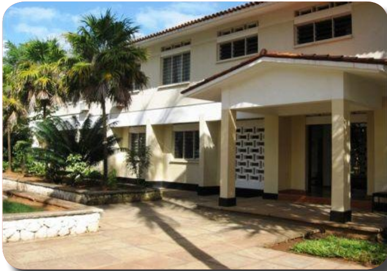
The Old Administration Block
